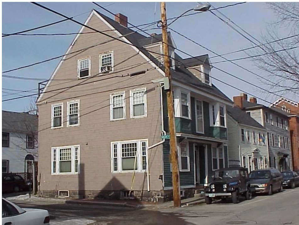
Figure 1 – Photograph of 20 Chapel Street circa 2001
