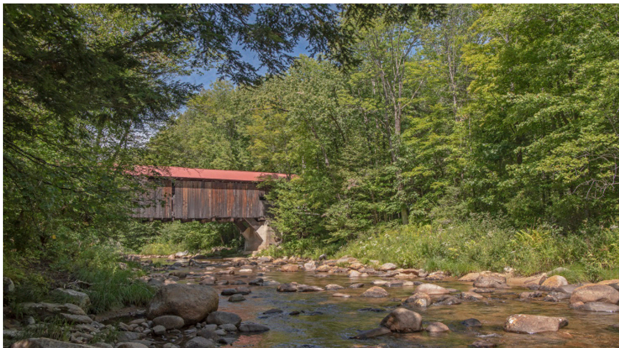
Durgin Bridge, Sandwich, NH
